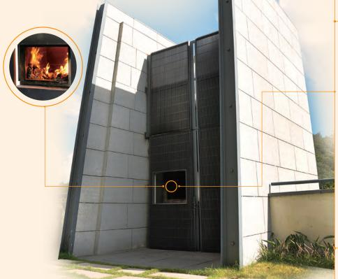
15個「清煙環保化寶爐」分別安裝於兩座大樓,減少燃燒冥鏹時所排放的黑煙。 15 environment-friendly furnaces, "Qing Yan" Smokeless Joss Paper Furnaces, were installed in these two premises to remove black smoke emissions from joss paper burning carried out by the public.
